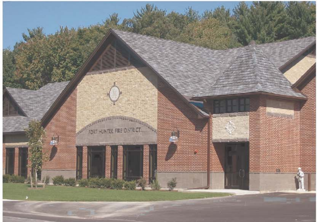
Photos courtesy of Richard E. Jones Associates
